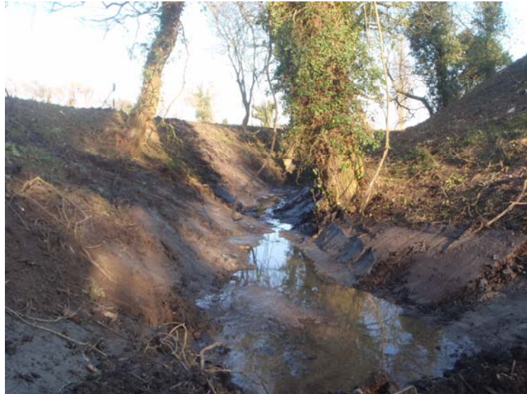
Plate 8. Motte ditch on the north-east side looking south-east after the removal of the later silts. The limit of the excavations were inside the original cut of the moat ditch in order to preserve evidence of its shape
