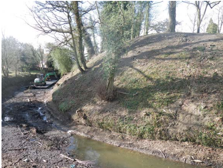
Plate 10. SE corner of the bailey bank and moat facing west. Note how the water action has eroded a channel at the base of the bank which was exposed when the water level was reduced
