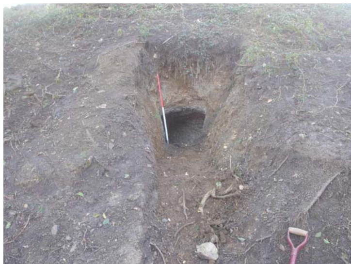
Plate 15. Modern, man-made, 'foxhole' burrowed into the east side of the motte at mid-height. The hole is accessed by a cutting excavated into the side of the mound and the hole extends 1-1.5m into its core
