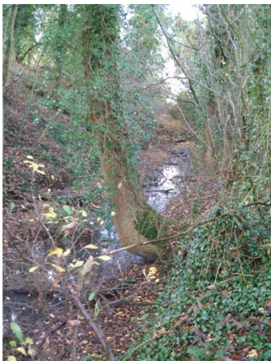
Plate 1. Bailey moat, choked and overgrown, on the east side of the castle facing north prior to the start of work
